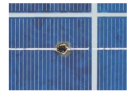
PV panel burned out by an arc discharge
