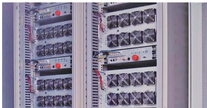
GBM power supply unit (charging/discharging control panel)
