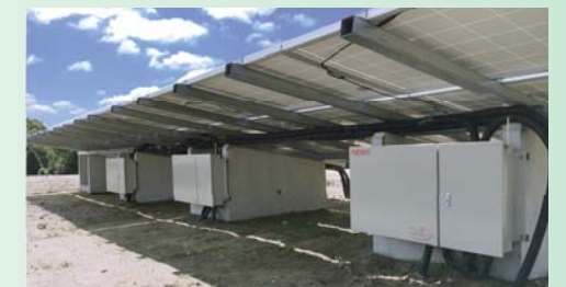
Example of PV Maximizer installation
