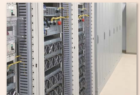
Interior installations in the container
