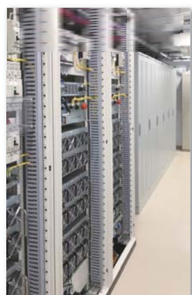
Interior installations in the container
