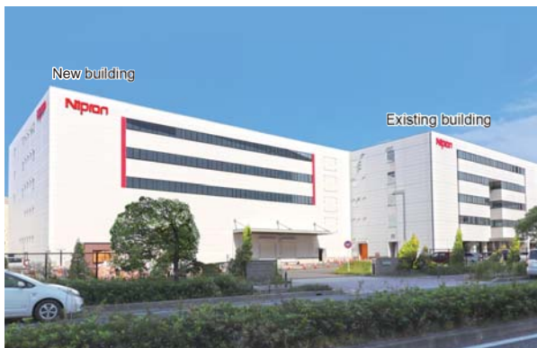
Head office/Hanshin Dream Factory (HDF)
