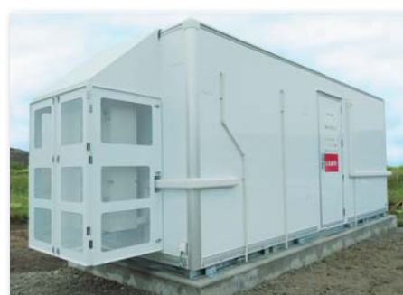
External view of the power storage system container
