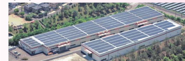
A power station at Yamakoh Co., Ltd.
