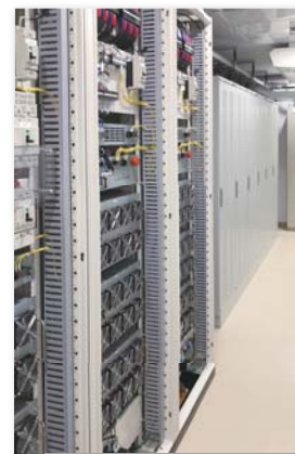
Interior view of installations in the container
