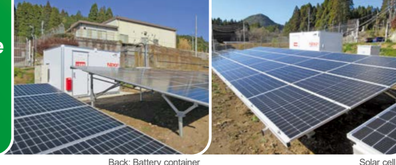
Back: Battery container
