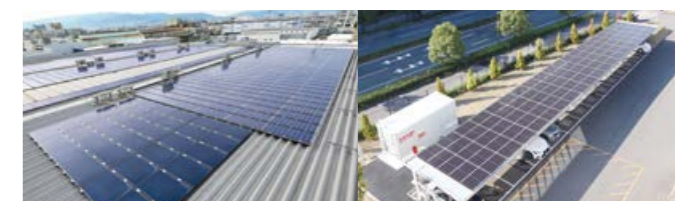
Head Office & Hanshin Factory
